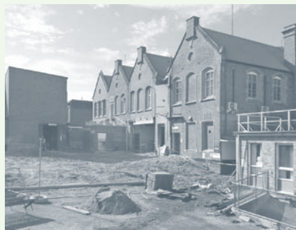
Hospital redevelopment works will include a second emergency theatre, a modern day surgery ward and recovery area, an improved front entrance and relocation and refurbishment of the accident and emergency department.
